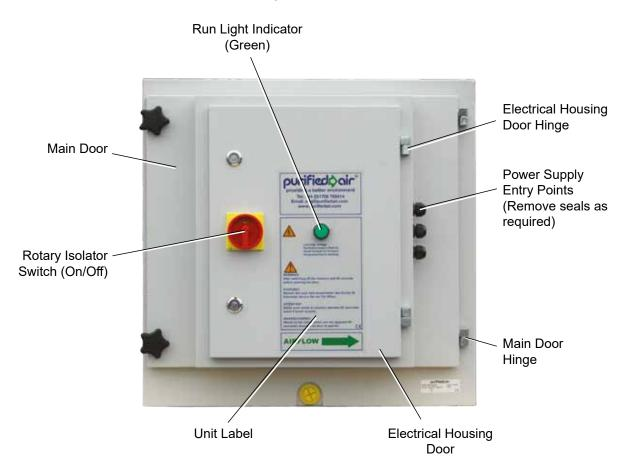
Figure 15 - Control Panel Components
